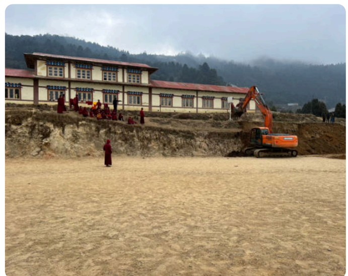
PLAYGROUND UNDER THE CONSTRUCTION
